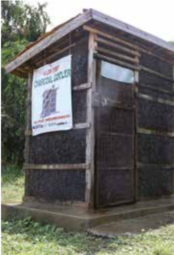
Prototype charcoal cooler developed at Makerere University.
